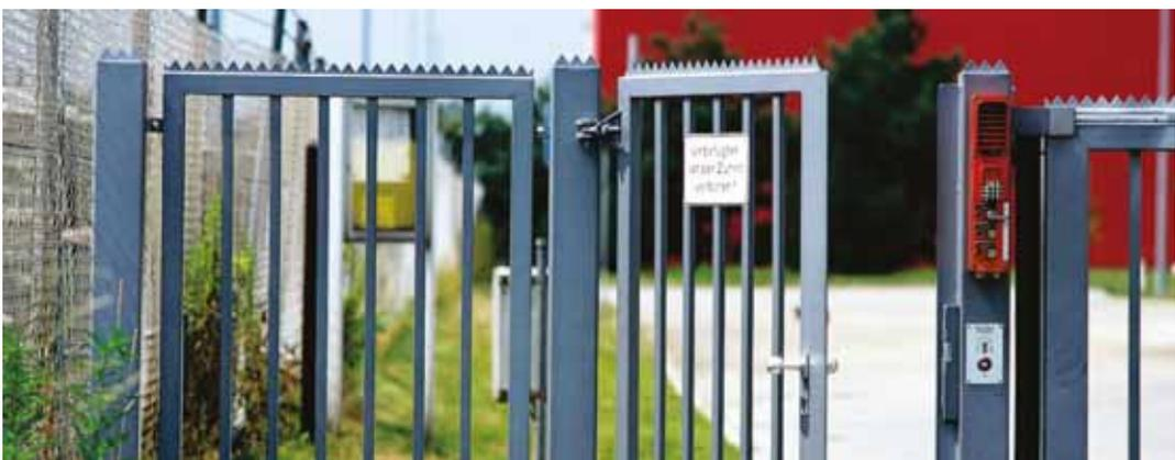
**Figure 7-14:** Serrated ledge as anti-climb guard
