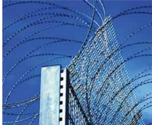
**Figure 7-15:** Combined anti-climb guard (expanded metal with coiled razor wire)
