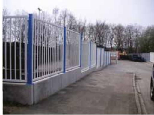
**Figure 7-9:** Front guard fence with floor plates
