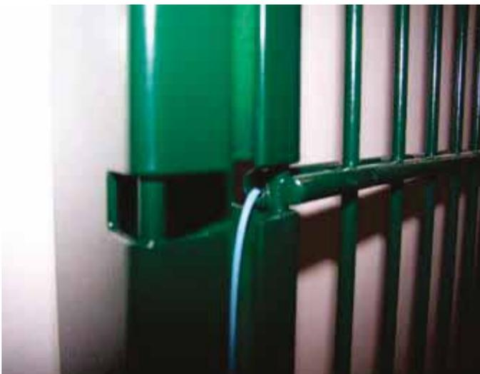
**Figure 8-2:** Detection fence with alarm wire inserted
