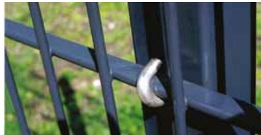
**Figure 7-7:** Bar grating fence with horizontal flat steel profile as endless fence with variable distances between posts
