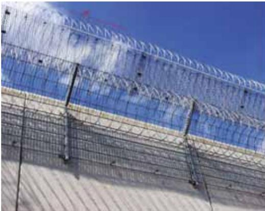
**Figure 7-12:** Razor wire, coiled with concertina effect (barrier belt)
