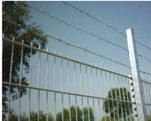
**Figure 7-13:** Classical barbed wire as extension of bar grating fence
