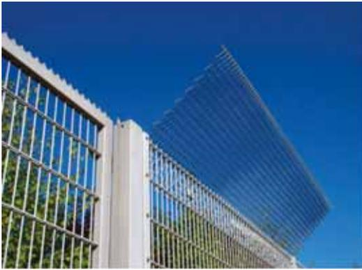
**Figure 7-10:** Flexible plate of expanded metal as anti-climb guard
