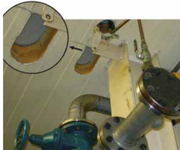
Fig. 6.05: example of an unprotected opening in a sandwich element with exposed installation material
