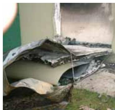
**Fig. 6.02:** Sandwich elements after a fire
